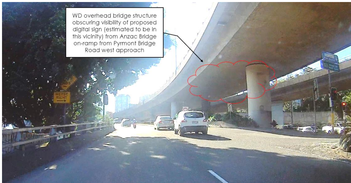
Figure 3.6: Anzac Bridge on-ramp from Pymont Bridge Road
